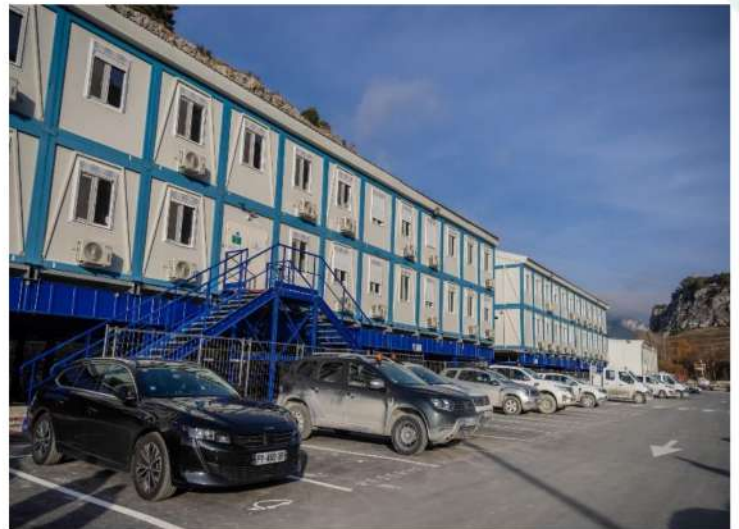
Base chantier Modane
